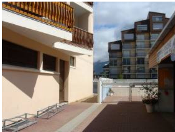
Building Entrance on left
