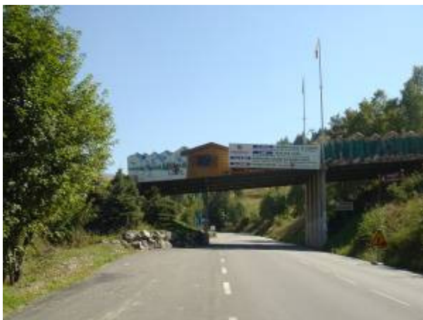
Bridge Over Main Road
