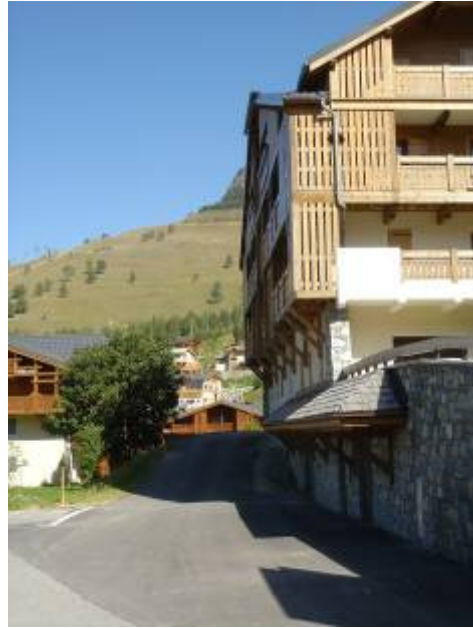
Driveway to left of building
